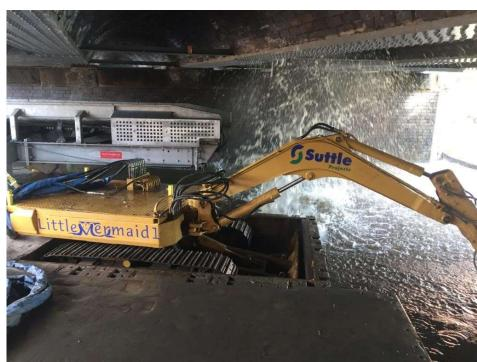
handgun, that was duly reported to local police. This made tracking of our excavator on the riverbed untenable, both in terms of entanglement and likely hydraulic leaks from metal punctures. We re-thought. Instead we used a recessed pontoon to create an ultra-low headroom floating digging device, incorporating the Mermaid beneath the bridge.
